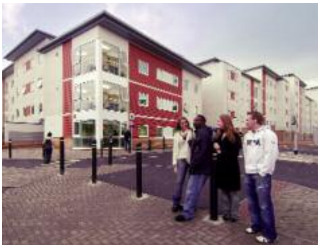
Talybont Court, the University's newest residence
